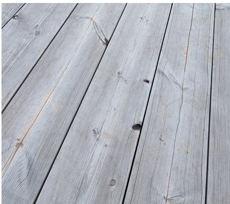
Untreated Lunawood decking (Thermo-pine) 2 years after installation. Small hairline cracks can be seen on the surface.
