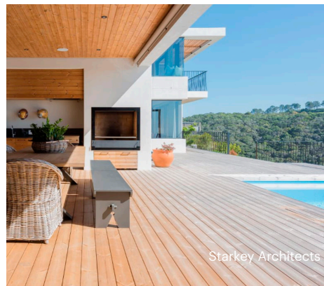
Terrace of a private home in South Africa. The decking in the sunny area has turned gray faster compared to the shaded area.
